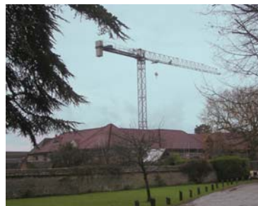
The 'La Verna' extension under construction
