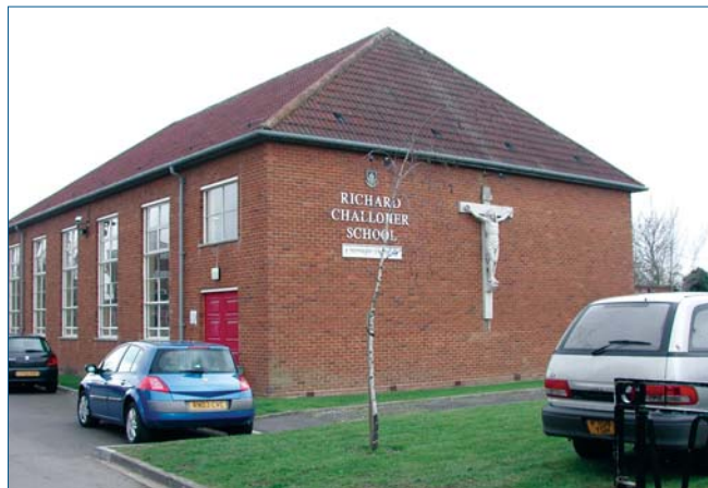
The Richard Challoner School, New Malden – where our Building Surveyors have been successfully winning DfES Capital Funding
