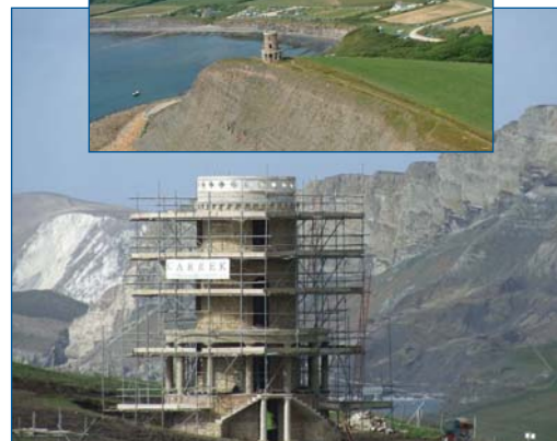
Clavell Tower, top, before relocation and bottom, under reconstruction
